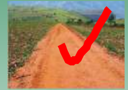
Well planned crest road contoured to limit erosion
