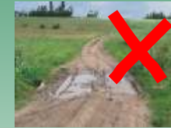
Poorly planned road through a wetland
